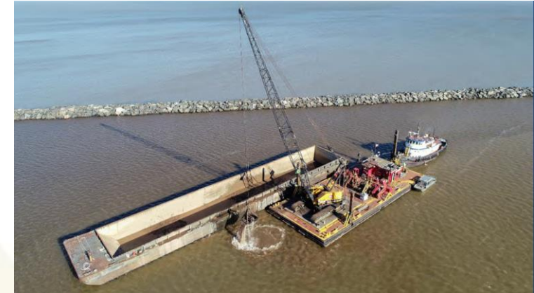
Minnesota Slip beneficial use dredging at Superior Entry
